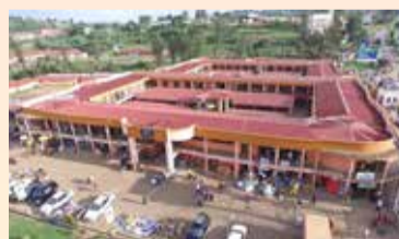
Mpanga Market constructed under MATIP-1 Project
